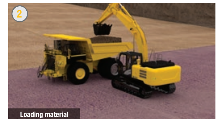
2 Loading material Loading equipment places the material in over-the-road trucks to haul it to offsite locations.
