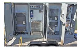
MOTOR STARTER PANEL. The motor starter panel provides options to configure a control system that best fits your application – whether that's a soft-start or VFD panel.
